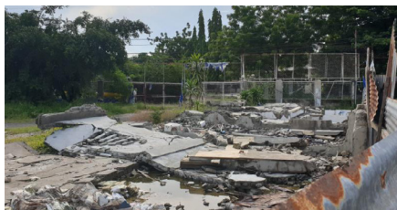
Pililia, Rizal Pre-Construction Phase
