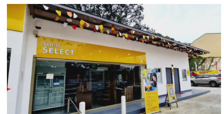
Tanay, Rizal Finished Construction
