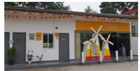
Pililia, Rizal Finished Construction
