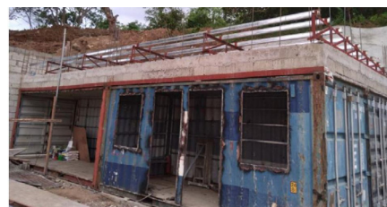
Tanay, Rizal Construction Phase
