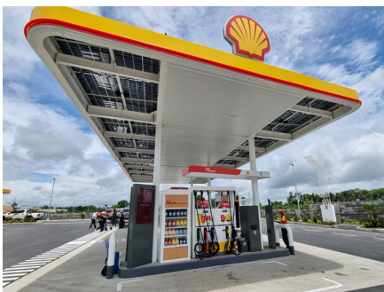
Solar panels on canopy roof and building eaves
